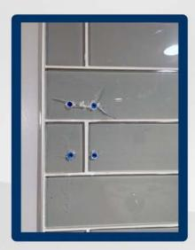
Glass tiles are increasingly popular, but should always be kept away from areas where hinges and hardware will be set. Drilling through glass tiles leads to cracked tiles no matter how careful one is. Choosing an alternate material for these areas, such as a complementary color of tile or marble, is the best way to eliminate this issue.
